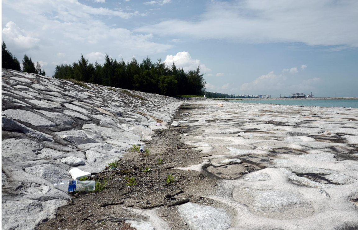
Figure 3.8 View of the rocky revetment at Tanjong Rhu on 23 Apr. 2021. Photo by author.
